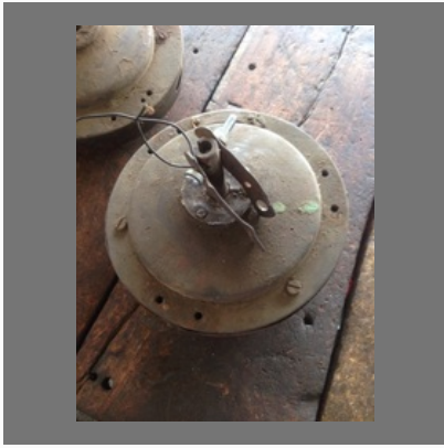
Ceiling Fans Repairing
