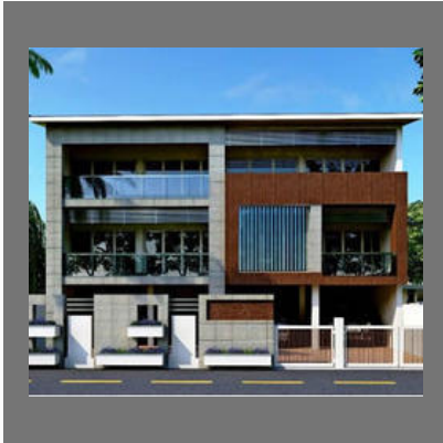
Villa Linavala Architectural Services
