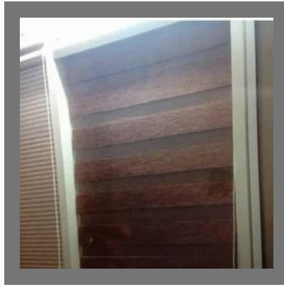
Aluminium Fabrication Work
