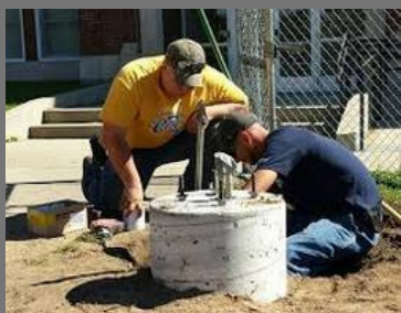
Underground Electrical Works
