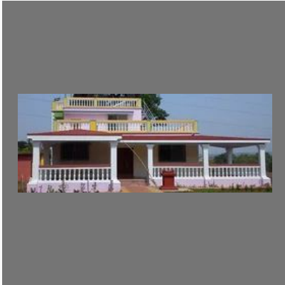
Cottage Construction Service
