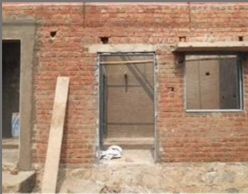
Shop Construction Service
