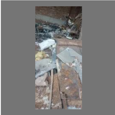
Iron Sheet Scrap
