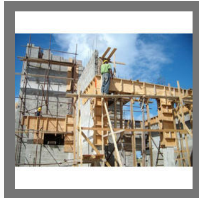
Civil Construction Service
