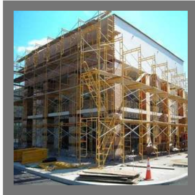
Commercial Construction Projects
