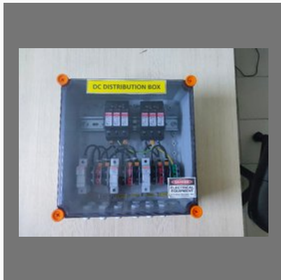
Solar DCDB Box 3 IN 3 OUT 2 SPD 1000 VDC FOR 11-16 KW
