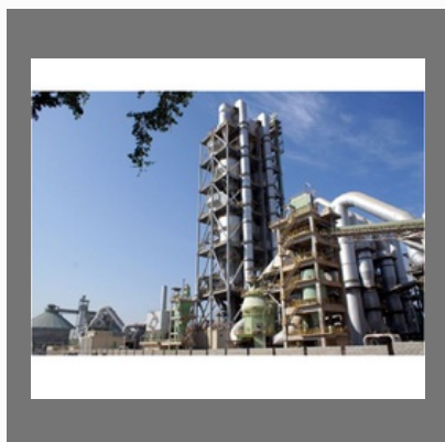
Rotary Kiln Cement Plant
