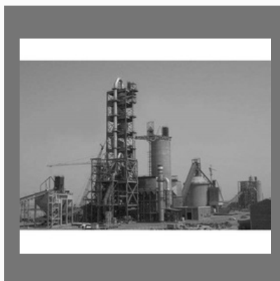
VSK Cement Plant
