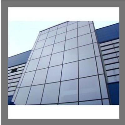
ACP Glass Glazing
