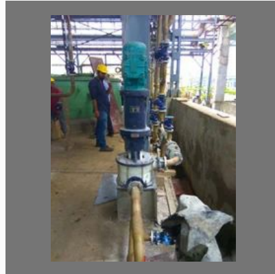
Vertical Glandless Pump Installation
