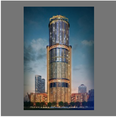
Hotel Building Construction Services
