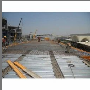
Roofing Sheet Installation Service
