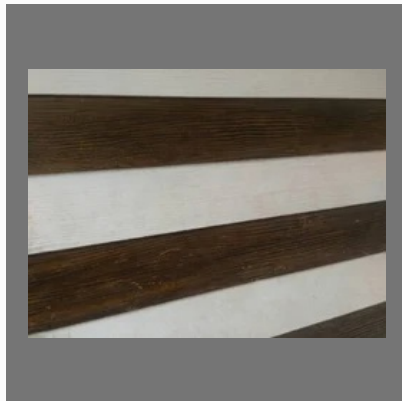
Multiple Ceiling Panels
