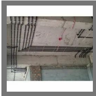
Wiring Installation Service
