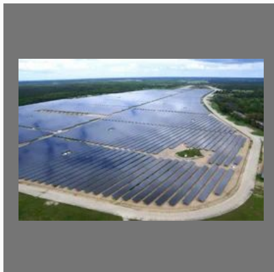
Solar Power Plant Installation
