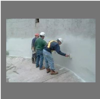
Water Tanks Waterproofing Services
