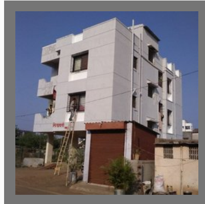
Exterior Wall Waterproofing Services
