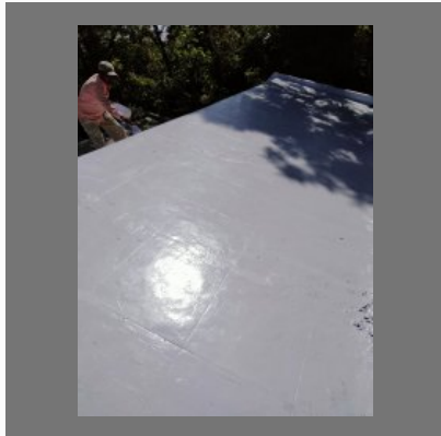
Terrace Waterproofing Coating Services
