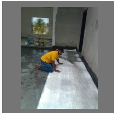
Bituminous Waterproofing Service
