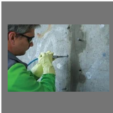
Injection Waterproofing Service
