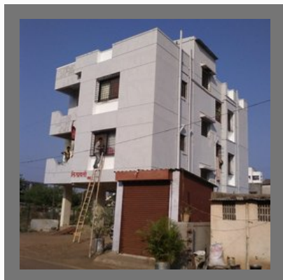
Building Cracks Repair Service
