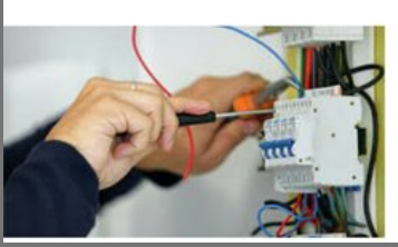
School Building Electricals Services
