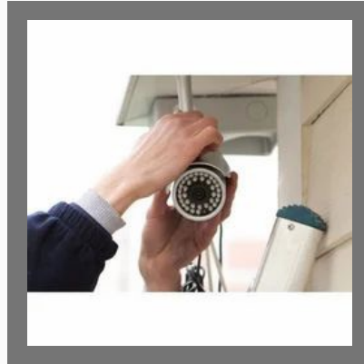
CCTV Camera Installation Service
