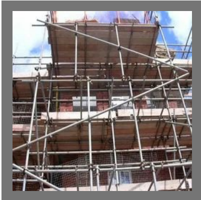
Mild Steel Scaffolding
