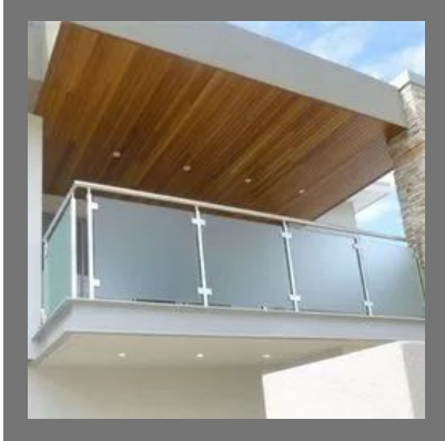
Railing Fabrication Work
