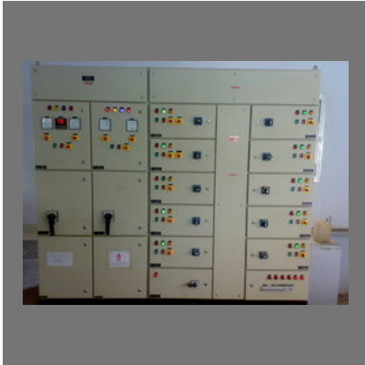
Motor Control Center Panel
