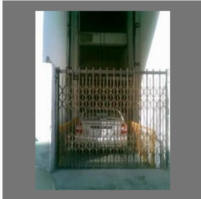
Mild Steel Car Elevator
