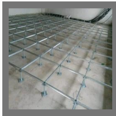
Installation Of False Flooring
