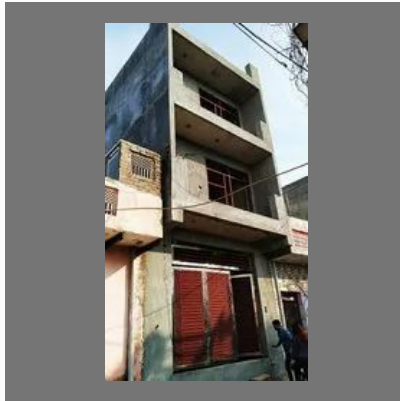
Flats Construction Services
