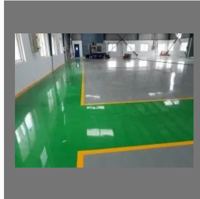
Anti Corrosive Epoxy Coating Service
