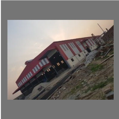
Steel Industrial Buildings
