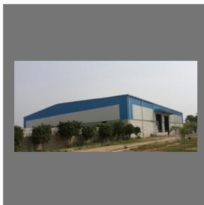
Industrial Steel Sheds
