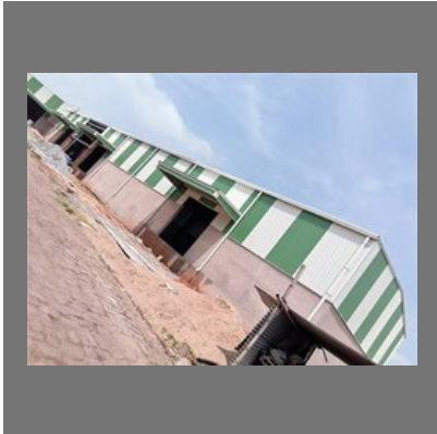
Prefabricated Factory Building Structure
