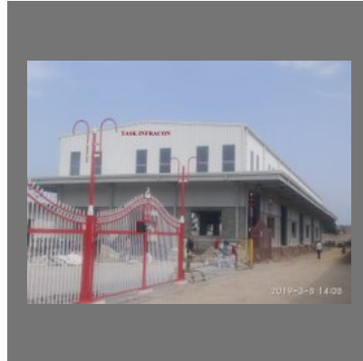
Peb Structural Shed
