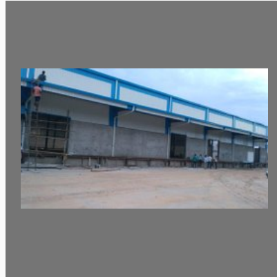
Industrial Pre Engineered Structure Services
