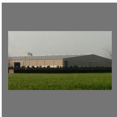
Warehouse Pre Engineered Structure Service
