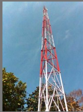
Internet Communication Tower
