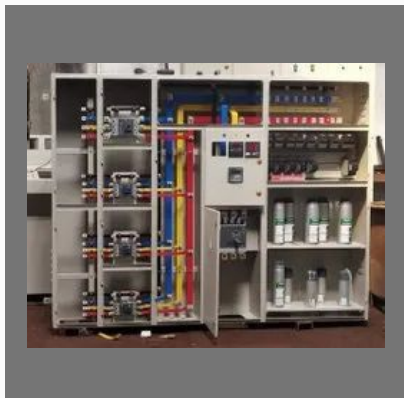
Electrical Items Repairing Services
