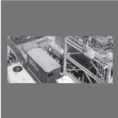
Deck Management System Solution
