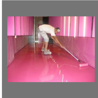
Epoxy Floor Screeding Service
