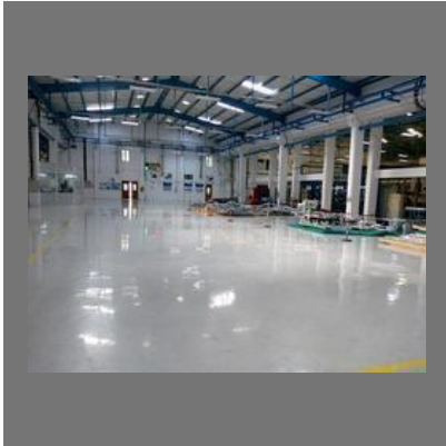
Factory Epoxy Flooring Service
