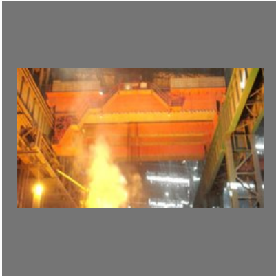
Steel Mill Duty Crane
