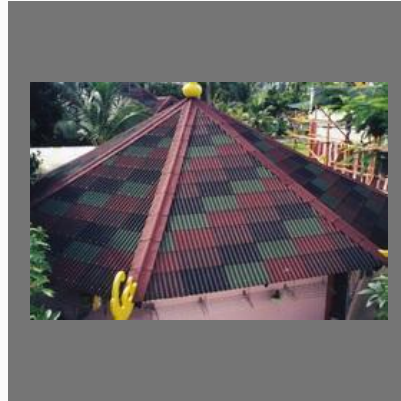
Residential Bungalow Roofing Sheet
