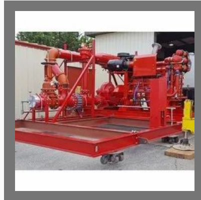
Fluid Handling Industrial Pump Skid
