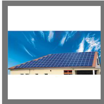
Solar Power Rooftop System
