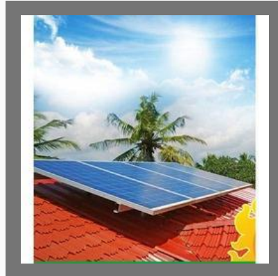
Solar Grid Tie Rooftop System
