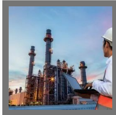
Building Management Solution Service
