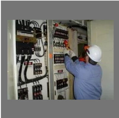
Industrial Electrical Wiring Work
