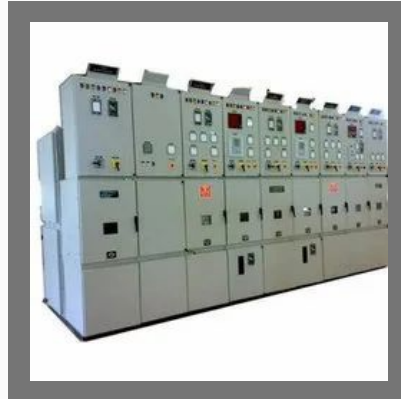
Industrial Electrical Contractor Works
