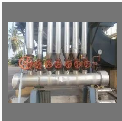
Steam Pipe Line Fabrication Services
