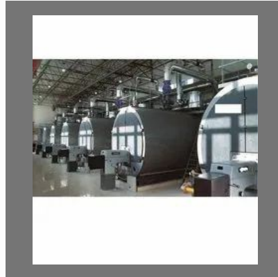
Boiler Erection Service
