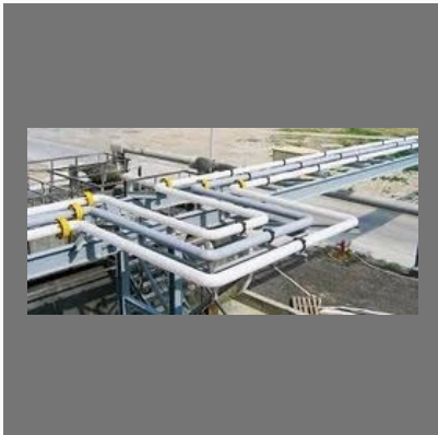
IBR Piping And IBR Boiler Repairing
