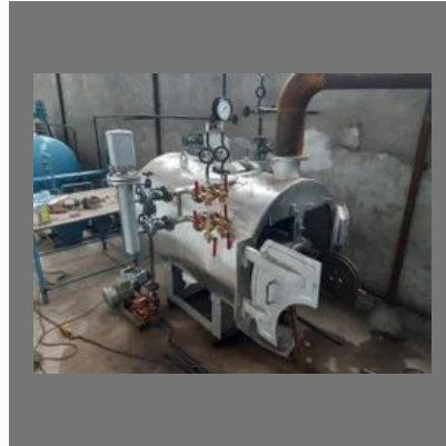
Horizontal Steam Boiler
