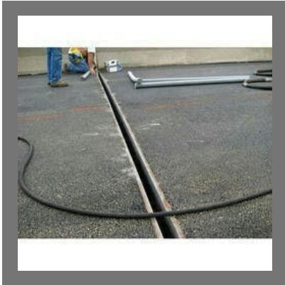
Expansion Joint Filling
