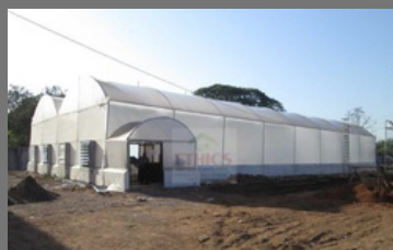
Forced Ventilation Greenhouse Services
