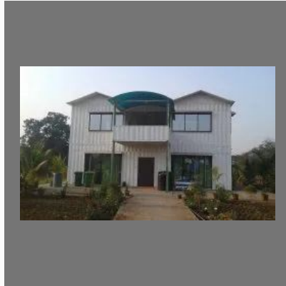
Construction Site Office Cabin
