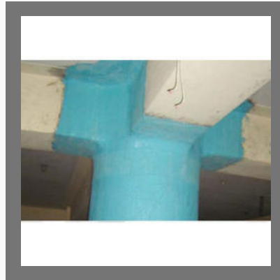
CFRP Wrapping Service
