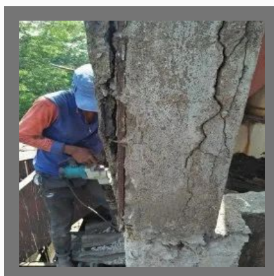
Structural Strengthening Work
