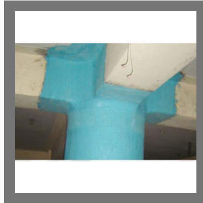
Glass Fiber Wrapping Contractors
