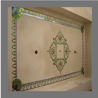
Interior Ceiling Work
