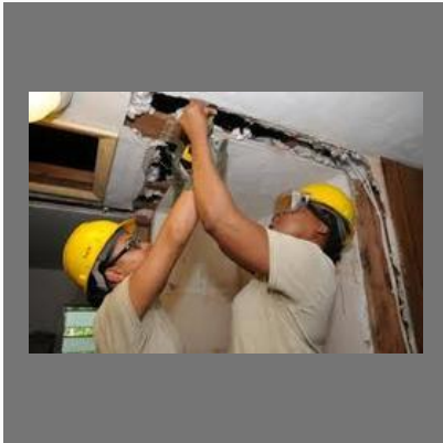
Carpentry And Masonry Jobs
