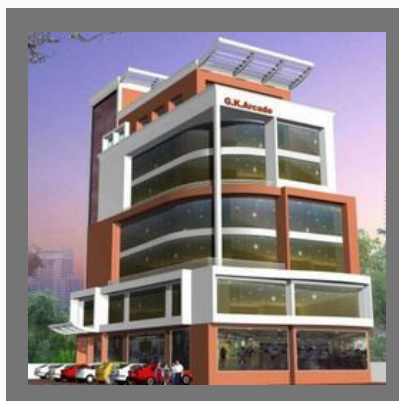
Commercial Complex Building
