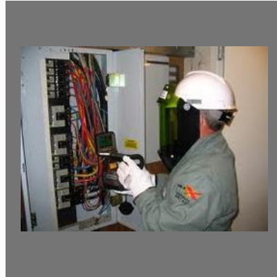
Electrical Maintenance Services
