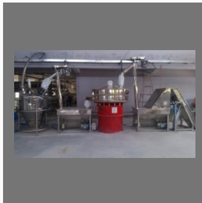
Flour Handling System
