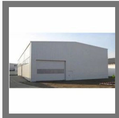
Prefabricated Steel Structure Warehouse
