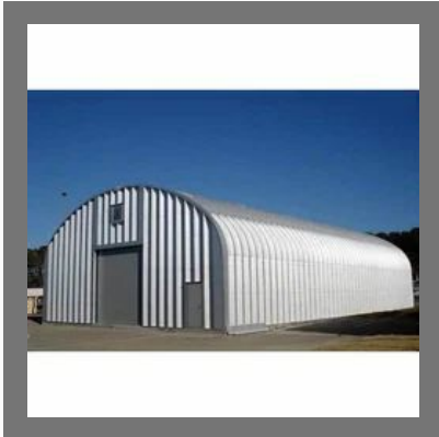
Steel Warehouse Building
