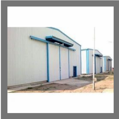
Prefabricated Warehouse Steel Shed
