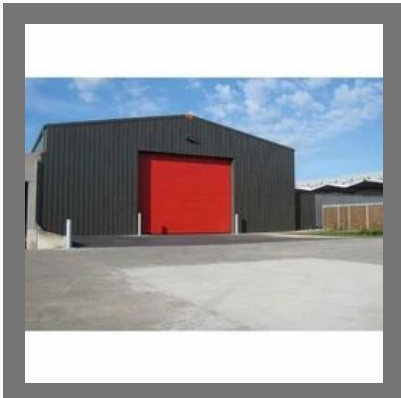
Modular Storage Building
