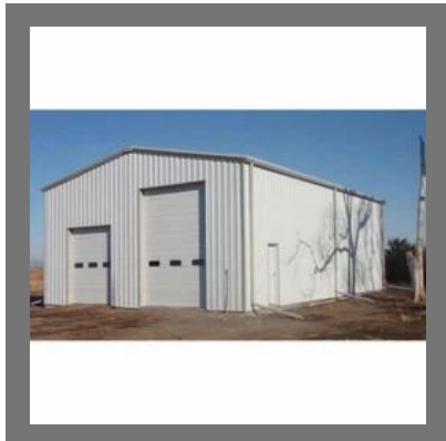
Mild Steel Structure Warehouse
