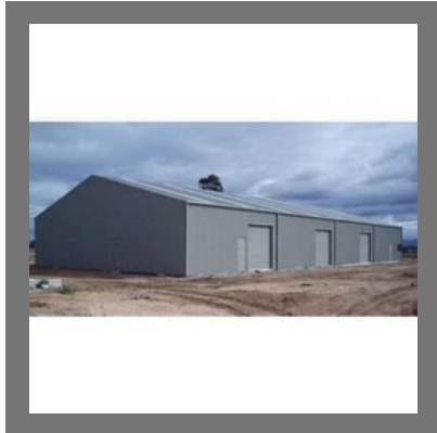
MS Structure Warehouse
