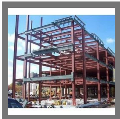
Structural Steel Fabrication
