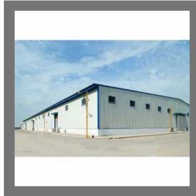
Prefabricated Factory Shed
