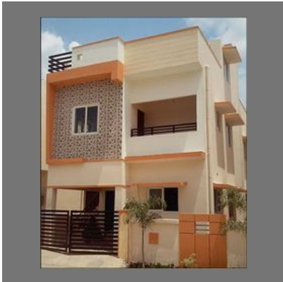
Luxury Villa Construction
