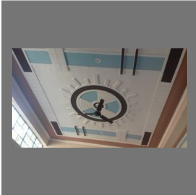
POP Ceiling Work & Design Saharanpur, Services
