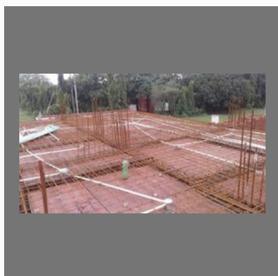
School Construction Services Saharanpur
