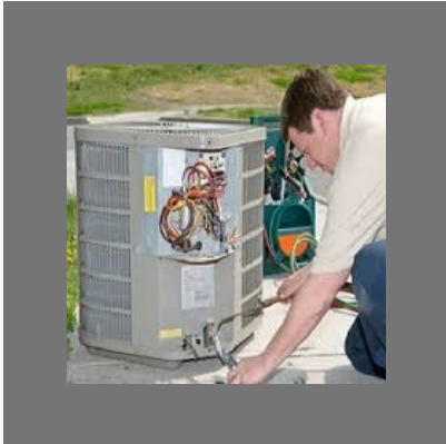
A.C. Repairing Service
