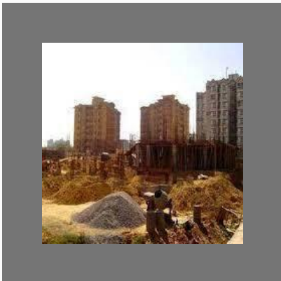
Residential Buildings Construction Service
